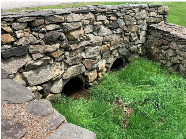
4 Brickyard – 1 (Drainage Course)
