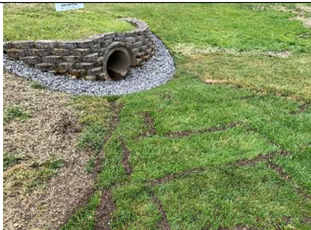
29 Gundalow -1 (Drainage Area)
