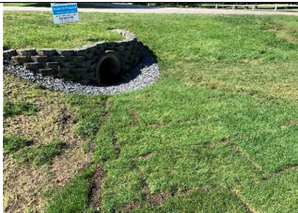
29 Gundalow -1 (Drainage Area)
