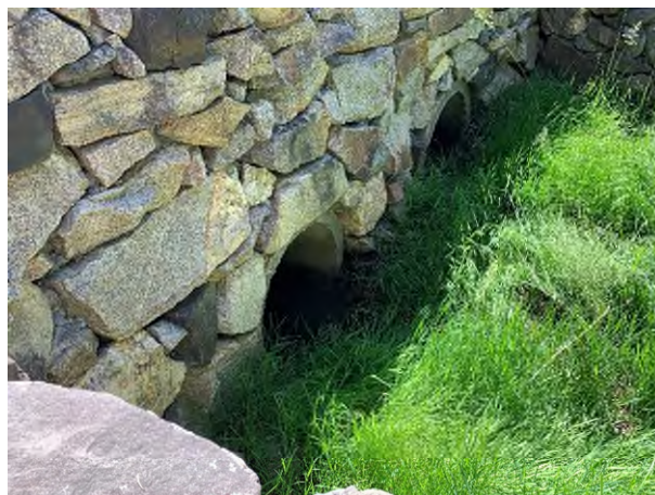
4 Brickyard - 1 (Drainage Course)
