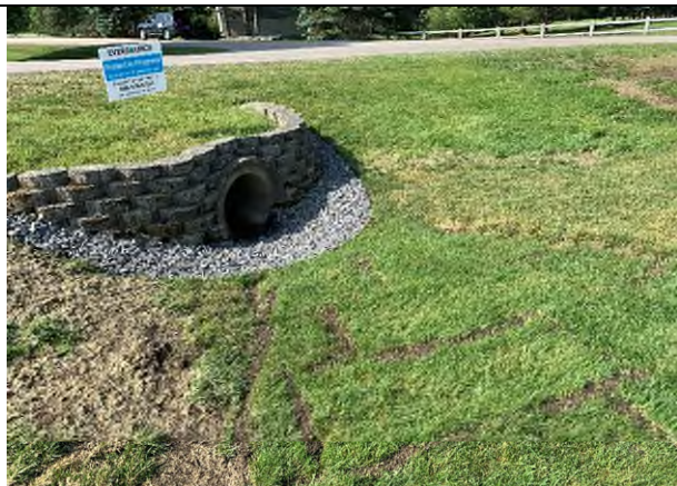
29 Gundalow -1 (Drainage Area)
