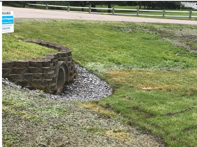
29 Gundalow -1 (Drainage Area)
