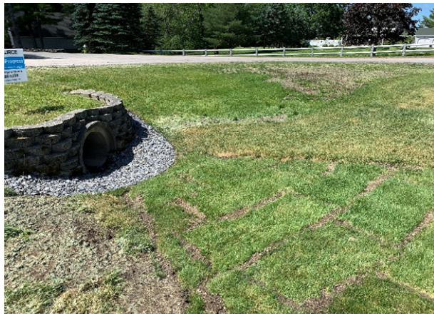
29 Gundalow -1 (Drainage Area)
