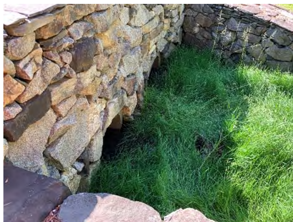
4 Brickyard Circle - 1 (Drainage Course)
