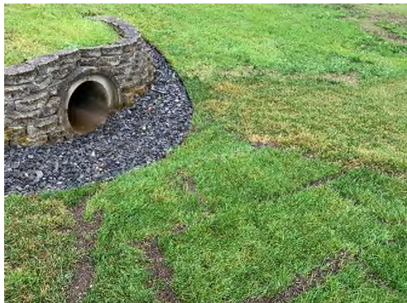
29 Gundalow -1 (Drainage Area)
