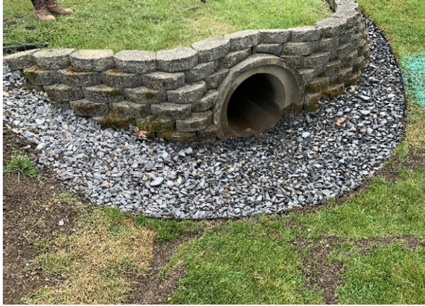
29 Gundalow -1 (Drainage Area)
